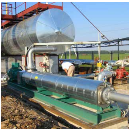
Transfer pump for crude oil in Russia
