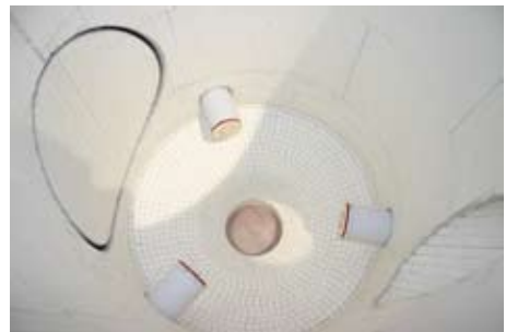
ceramic tile lined grinding chamber
